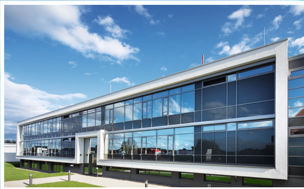
Company headquarters of Nabaltec AG, Schwandorf
